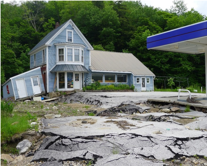
Blackies Deli in Bridgewater, Vermont was one of many local businesses that had significant damage after Hurricane Irene. The deli was demolished in 2014 and the site will remain open space. Credit: TRORC.
