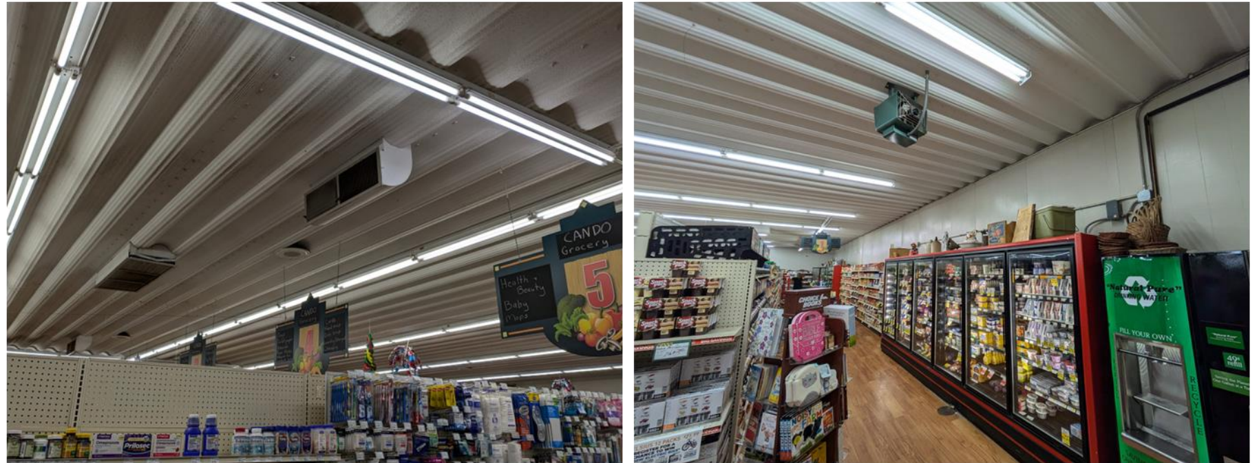
Cando Grocery HVAC replacement
